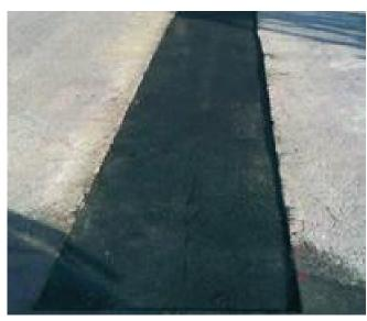
Fig. 2 - The cables are protected by concrete prior to further asphalt arrangement.
