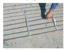
Protect the heating cables against excessive use of rakes, shovels, vibrators and rollers.
