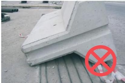
The elements and especially the connection must be protected from stress and strain.
