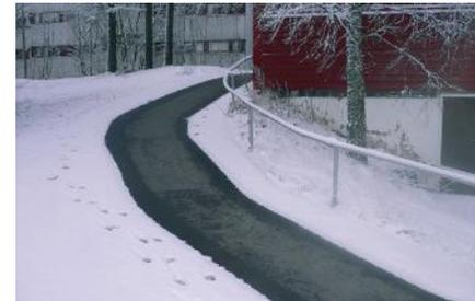
The element should be temperature controlled and not operate at ambient temperature higher than 10 °C in outdoor applications.
