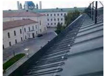
5. The selected cable should work as integrated part of an installation in the gutter and drain pipe, so connect it to the same control, e.g. DEVIreg™ 850.
