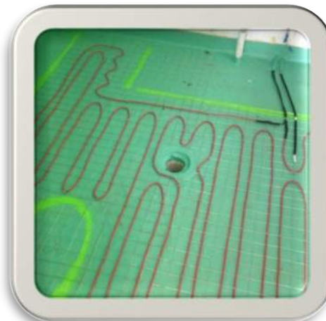
Wet Area on mesh on a membrane
